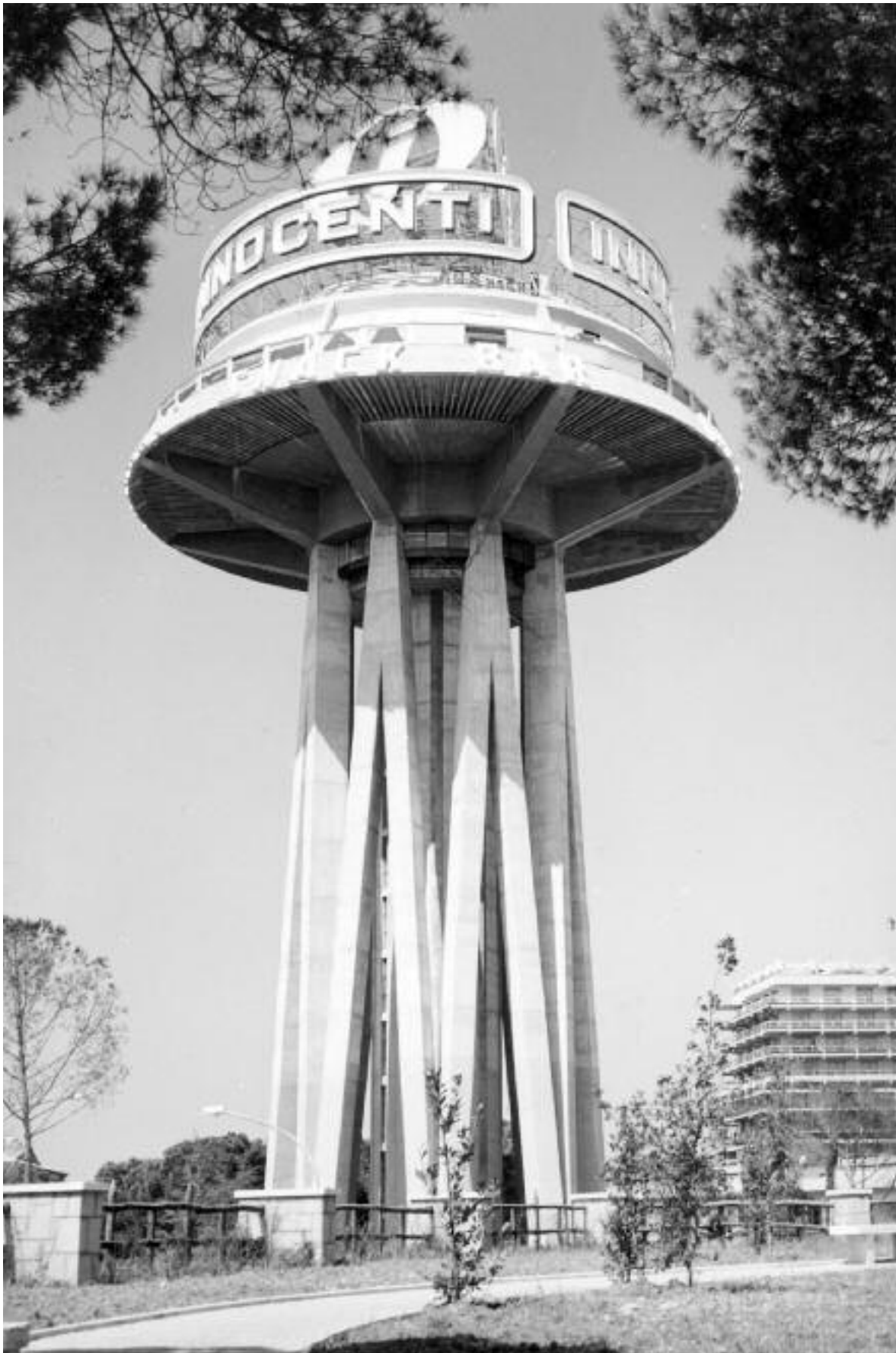
Lazio, Rome – Water tower in EUR
